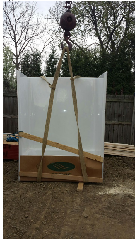
Figure 8.12 – Bathtub hooked to crane
