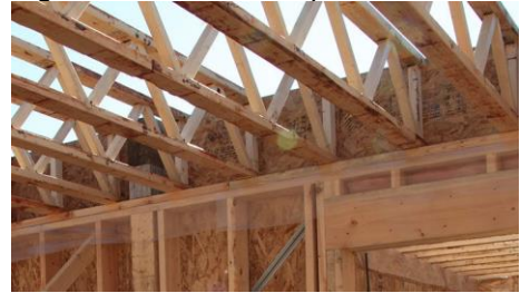
Figure 4.1 – Triforce Open Web Joists
