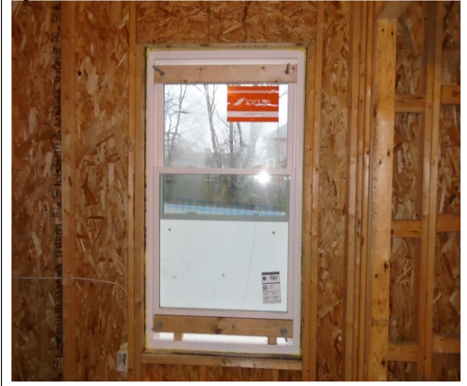
Figure 12.7 – Lexan over the windows
