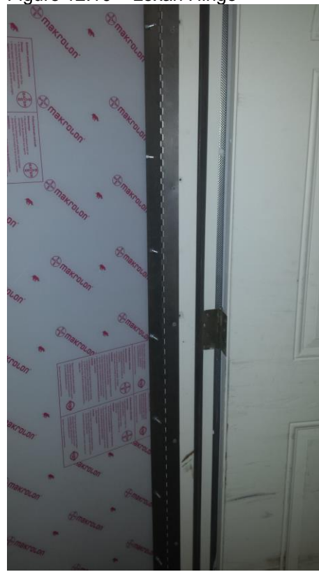
Figure 12.10 – Lexan Hinge
