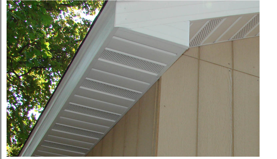
Figure 16.11 – Soffit panels
