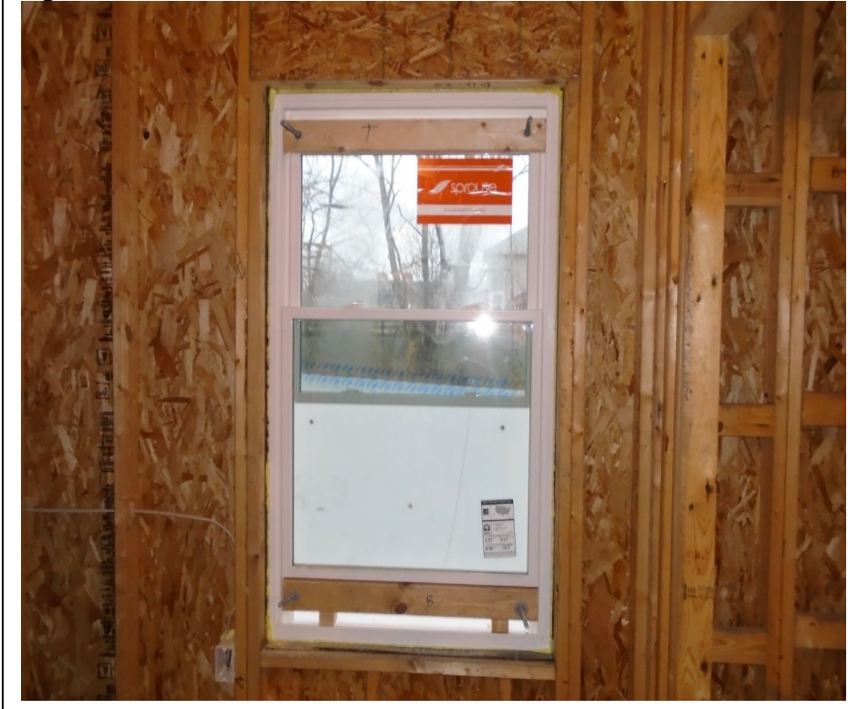
Figure 12.7 – Lexan over the windows
